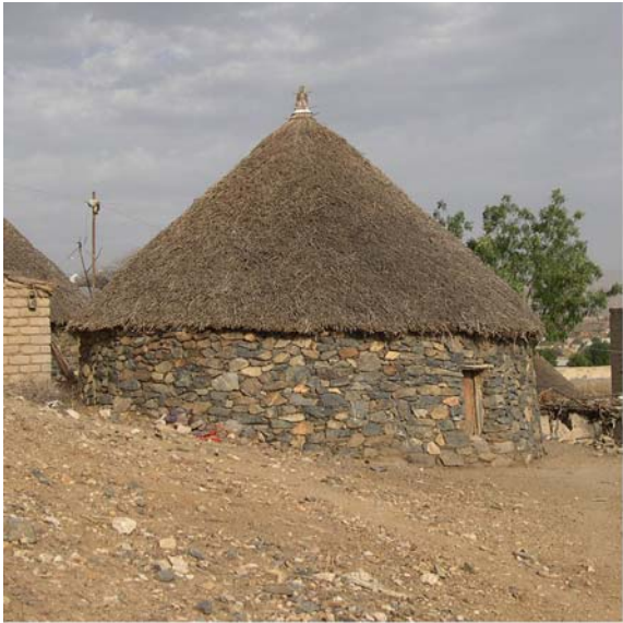
Asmara (Eritrea): tukuls made of stones (a) and made of rammed earth blocks (b)
